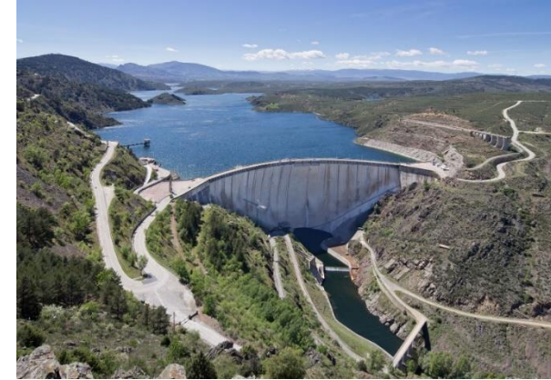
El Atazar Dam in Spain
